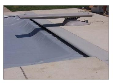
Finally, add the magnet to the tail end of the cover's webbing only when THE COVER IS IN THE CLOSED POSITION. 6-8" back from the guide, cut a slot in the webbing from the vinyl to the rope. Insert the magnet into the webbing and 1" past the center of the guide. This will stop the cover in it's current position. Now open and close the cover as needed. If adjustment is needed, adjust the knot & rope length. Congratulations! You're Done!
