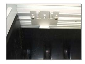
With (2) 3/8" x 3/4" bolts, install the motor end and opposite end mounting brackets into the lowest set of holes, preparing for the AutoGuard unit.
