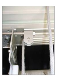
Slide the track into the coping. Be aware and keep the track from going into the pool. The pulley should be to the end of the encapsulation and the track should be ¾" into the box. THEN add the rubber wedge UNDERNEATH the track. This will hold the track in place. Continue to pull the rope around the opposite pulley and across the back of the polybox – leaving the rope by the motor end.
