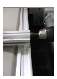
Now we will cut the track length. Measure the encapsulation (allowing for the end track pulley assembly see picture 1 above) PLUS the track must come <sup>3</sup>/<sub>4</sub>" past the inside of the coping and into the box end (see picture 2).
