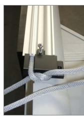
Unroll the vinyl from Left to Right. Pull the rope from through the correct guide, THEN pinch the rope thru the poolside of the track and pull to the end of the track. Next (picture 3) take the pulley around the pulley housing and thru the back channel of the track. Pull the track pieces together & tie the rope into a knot. This will make the track easier to slide into the coping.
